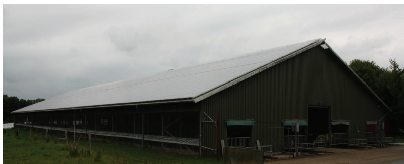
Fig. 1. Outside view of the investigated barn
